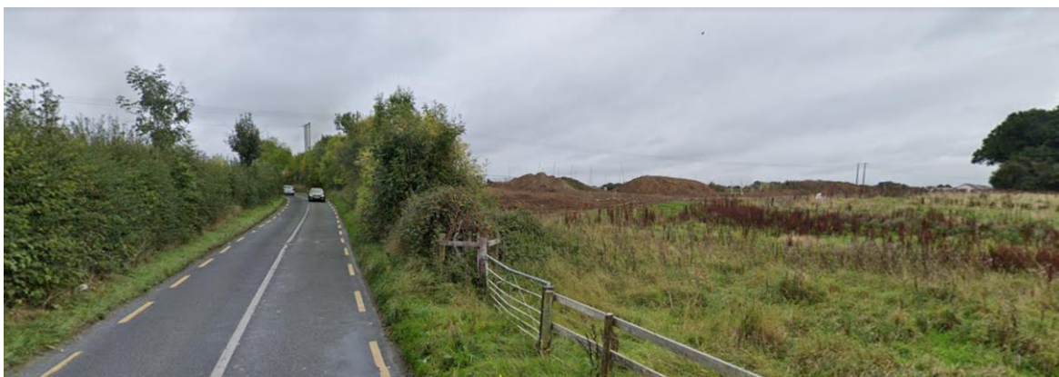
Figure 2.2: View looking East along Standhouse Road with the construction works for the road evident to the right of the image. (Source: Google Streetview, 2021)
