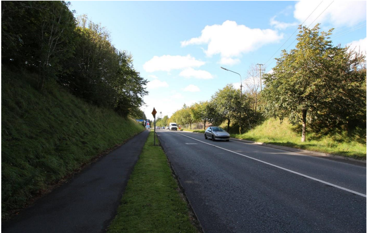
View 2 - Existing view from R445 towards the M7 Motorway interchange.
