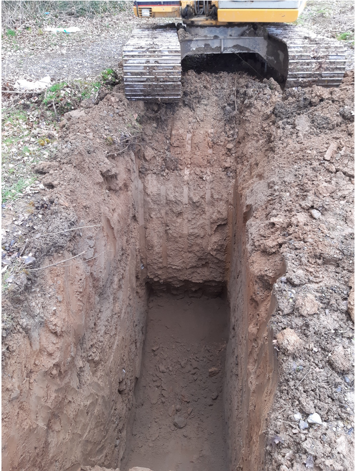
TP106 – Sidewall View
