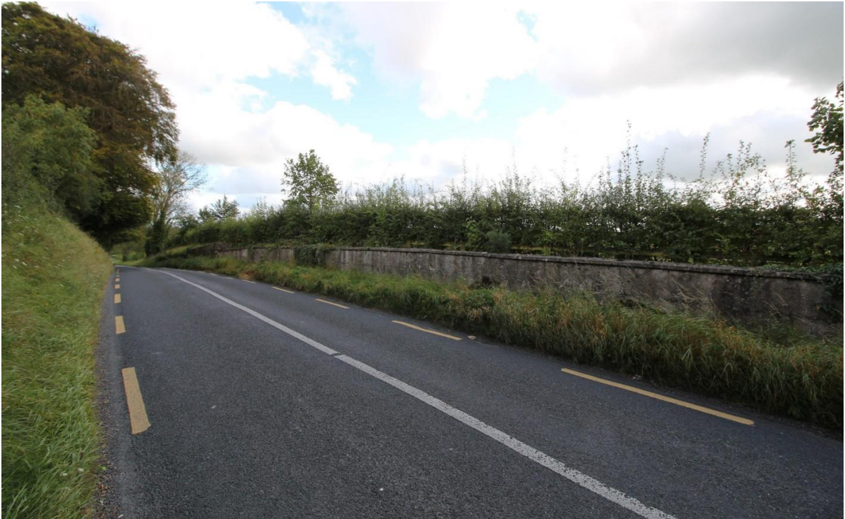
View 6 - Existing view from Strandhouse Road.
