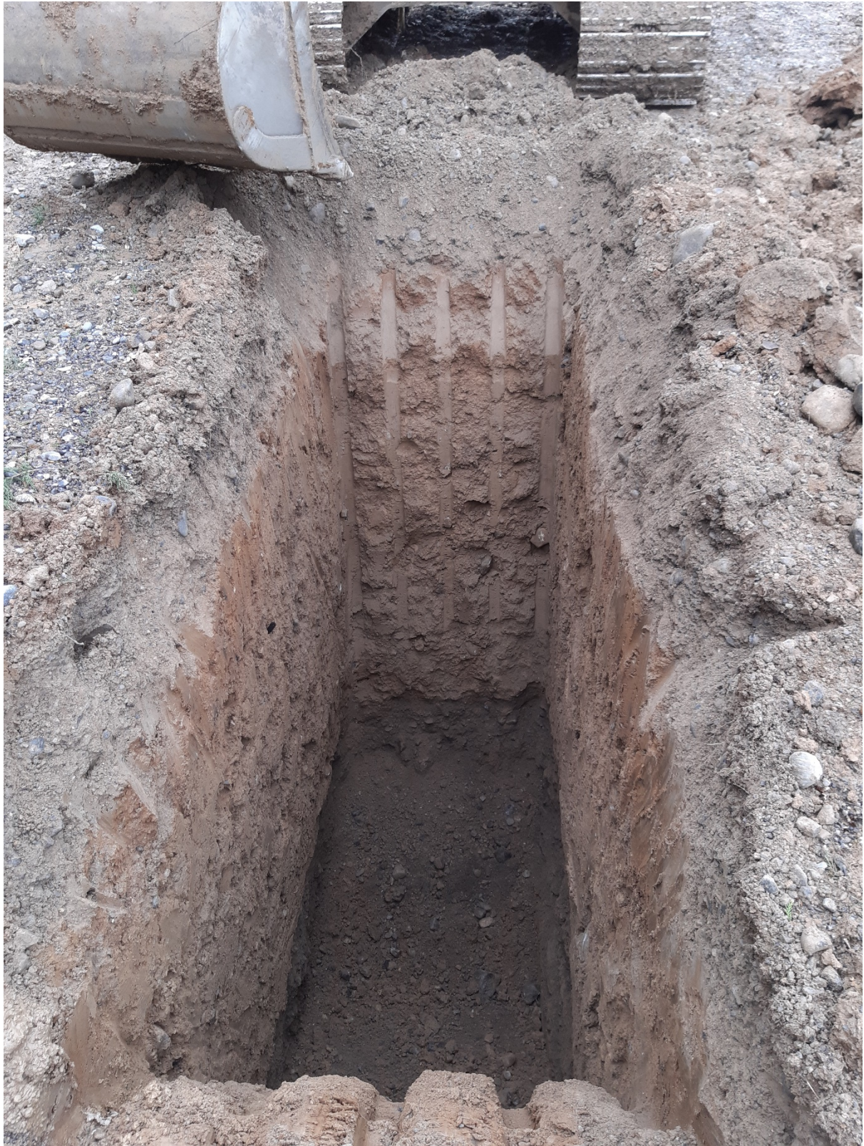
TP105 – Sidewall View
