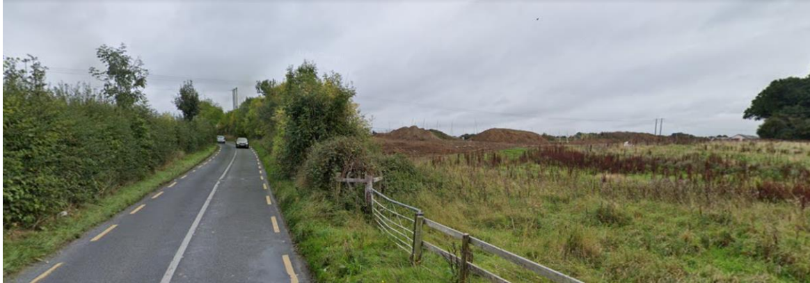
View looking East along Standhouse Road with the construction works for the road evident to the right of the image
