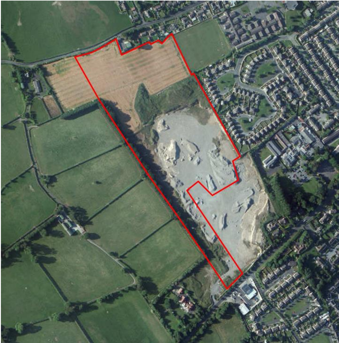
Figure 6.1: Aerial Image of the Proposed Development Site Illustrating the Extent of Previous Excavation on the Site;
