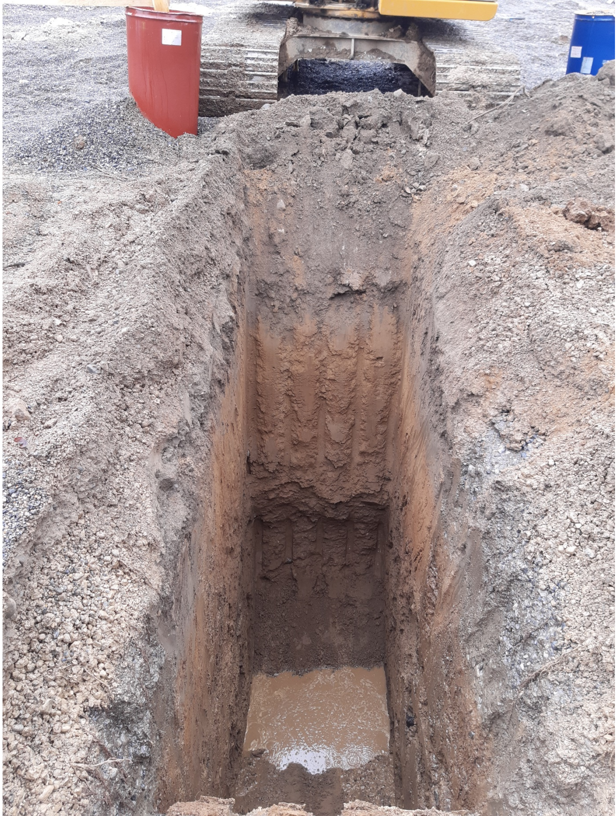
TP104 – Sidewall View
