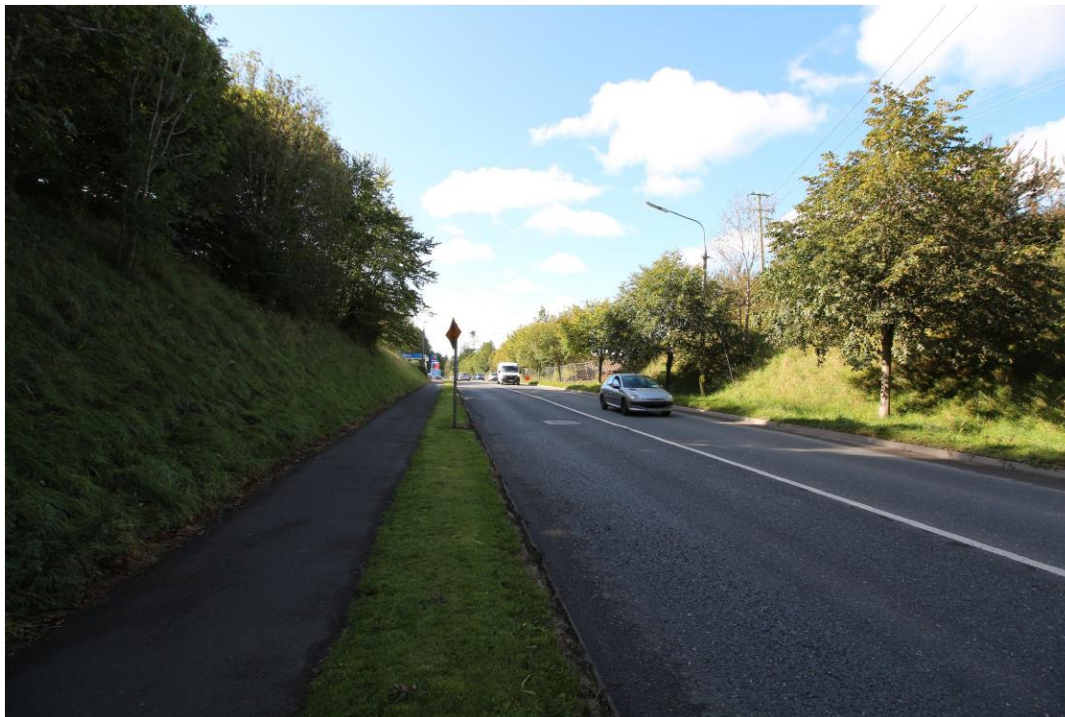
Figure 2.5: View looking south west along the R445 with berm at site entrance on the right. (Source: GNet3D, 2020)
