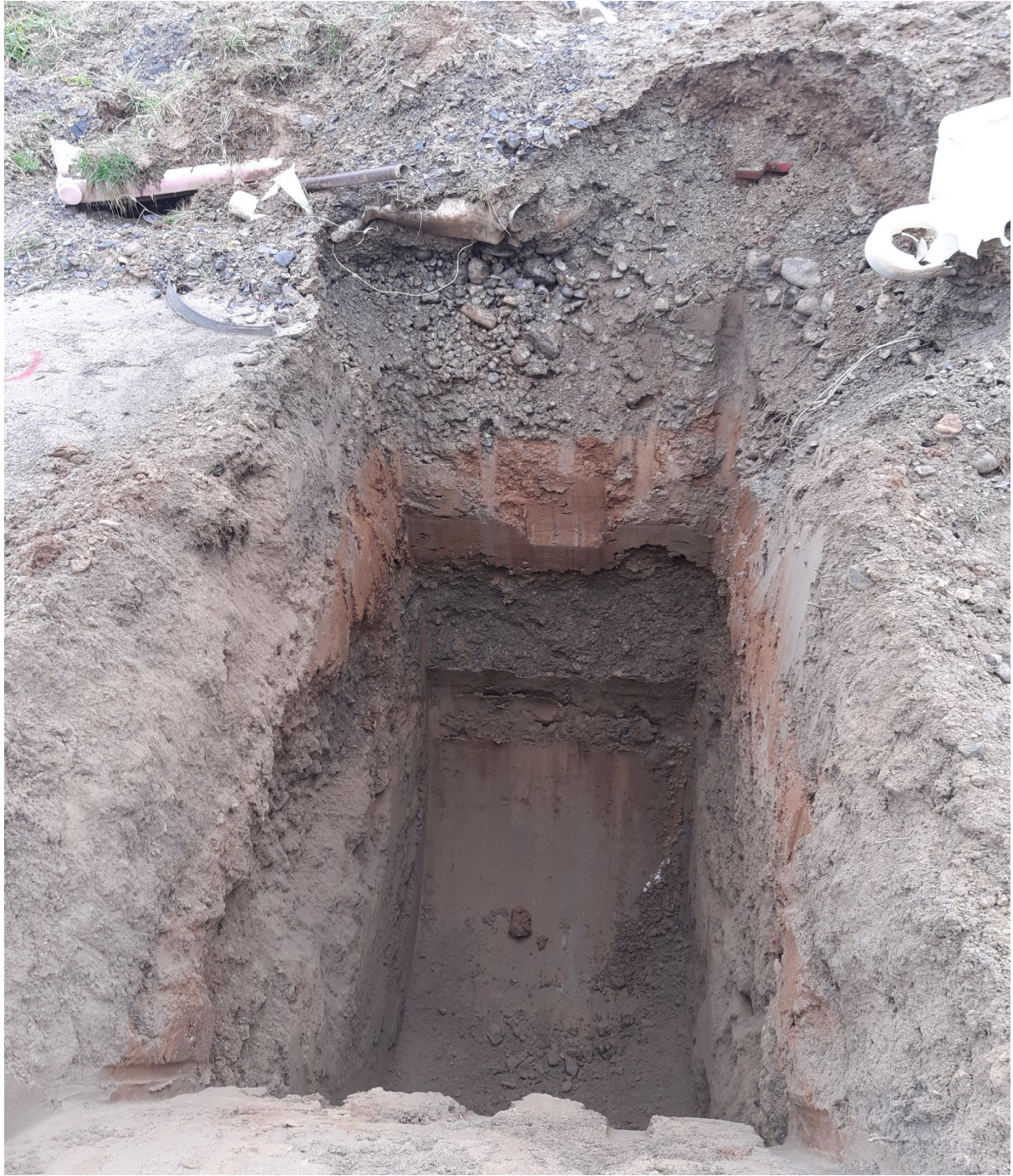
TP 102 – Sidewall View
