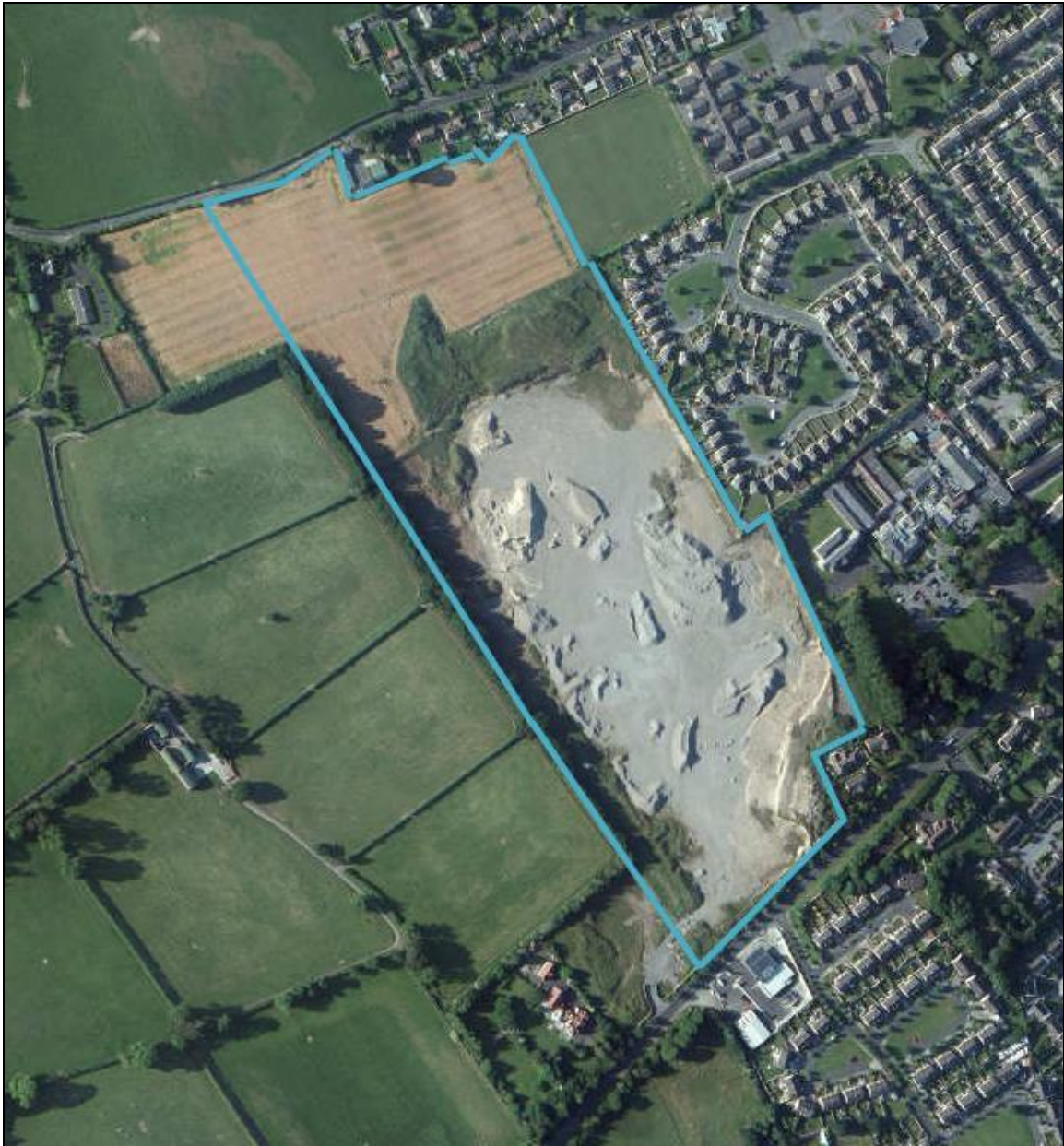
Plate 11.1 Aerial View of Overall Site – as existing
